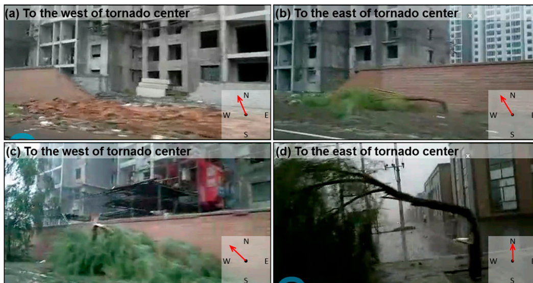
FIG. 7. Photographs of the fallen trees in Fig. 1f north of a west–east-oriented road on the southern edge of XDFZ, in which the lowercase letters correspond to different panels in this figure. The (a) western and (b) eastern ends of the downed wall. (c) As in (a), but \sim 20 m to the west with an eastward fallen tree. Shown in (b) is a westward fallen tree near the eastern edge of the downed wall. (d) As in (b), but \sim 30 m to the east, also showing a westward fallen tree. The red arrows in the bottom-right corner denote the direction that the photographer was facing. The pictures were snapshots from a video provided by Youku.com.
